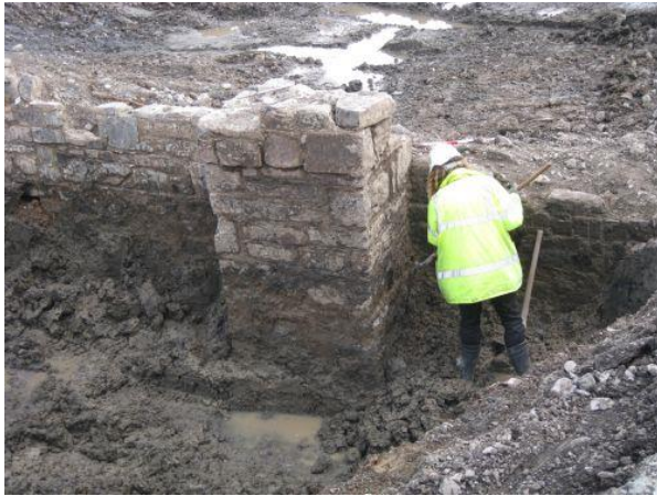
Figure 8: Cleaning newly exposed buttresses and retaining walls, Broadstone Harbour (Transport Infrastructure Ireland)
