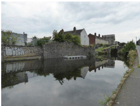
Figure 12: View from north-east of the Royal Canal 5th Level 6th Lock Gate and historic MGWR bridge abutment (Alastair Coey Architects)
