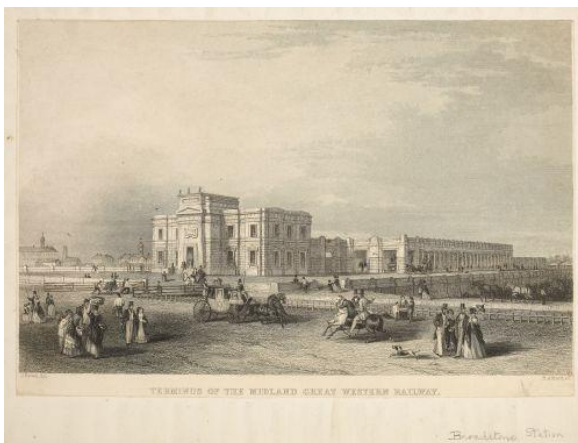
Figure 4: Terminus of the Midland Great Western Railway' at Broadstone by Henry Adlard (1828-1869). Note presence of Mallet's 'Insistent Pontoon Bridge' crossing the Royal Canal. © National Library of Ireland
