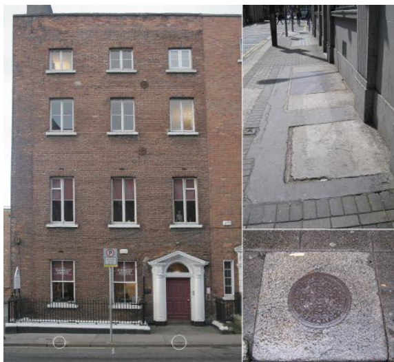
Figure 15: Typical Georgian building on 43 Dominick Street. Note insulating passage to fore, and coal hole covers parallel to street kerb (Left; Archaeology and Built Heritage); example of partially infilled lightwells/keg drops on Marlborough Street (Top right); example of coal hole cover with granite surround (Bottom right, Archaeology and Built Heritage Ltd)
