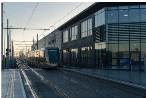
Figure 5: Luas terminus at Broombridge Hamilton Depot (Transport Infrastructure Ireland)
