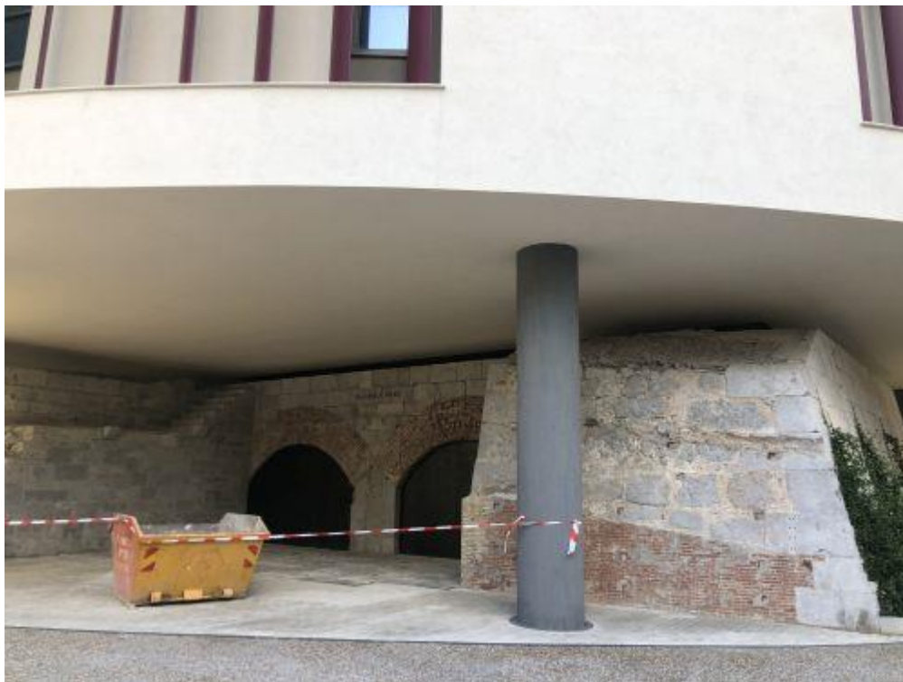
Figure 5: The Old Mole Head in Gibraltar (United Kingdom). In use until the end of the 19th century, it became absorbed by the city and somehow protected after the construction of a new secondary school over it. The creative solution in a place lacking construction surface would not be very satisfying elsewhere, but seems good enough under the circumstances of Gibraltar. Photo by the author
