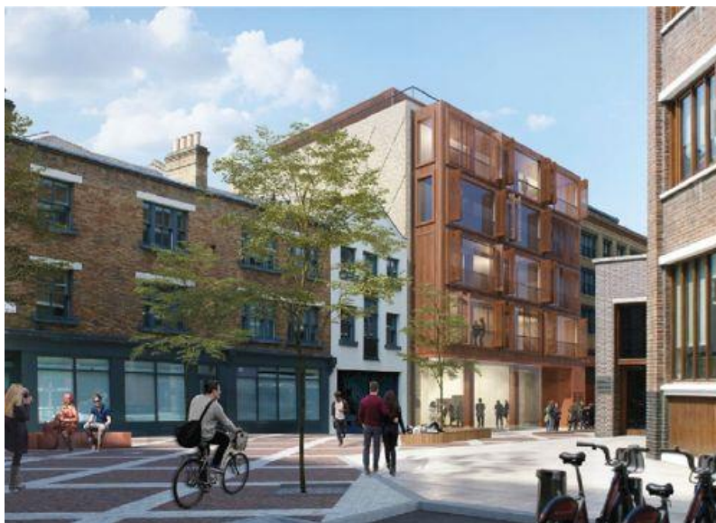
Figure 6: Exterior of 'The Box Office' development. © Gallus Studio
