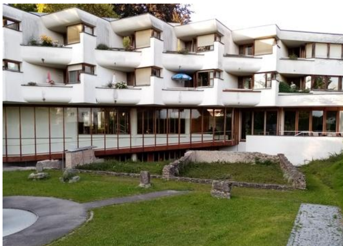
Figure 4: Remains of Brigantium 's middle imperial 'traders' quarter' (building 23), partially conserved inside and outside of the retirement home Tschermakgarten, an architecturally remarkable building erected between 1977 and 1979 (source: A. Picker).
