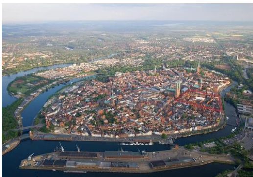
Figure 1: An aerial view of the Hanse city of Lübeck from the north-west, showcasing the island layout and the seven iconic church towers. Marked in red, below the two towers of St Mary's Church, lies the Founding Quarter, the historic area now undergoing redevelopment to blend medieval heritage with modern urban planning (© Hansestadt Lübeck, Abteilung Archäologie).
