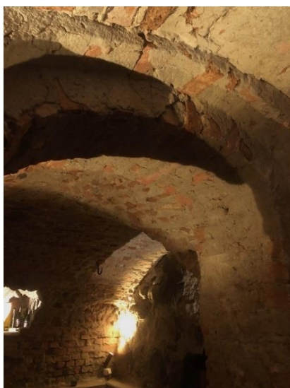
Figure 3: The preserved cellars of masonry houses from the early modern period on the premises of the Tårget restaurant, Turku, Finland. If discovered as ruins during an excavation, they would have been considered archaeological heritage and documented accordingly. In this condition and location, they have been considered built heritage without archaeological interest. Applying a holistic approach to urban archaeology, these would have
